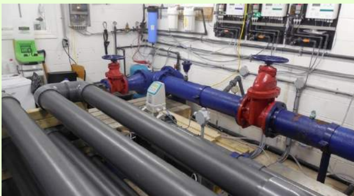
Sunnyside's new hydrogen peroxide-based water treatment system. Photo credit: Robert Snook.
