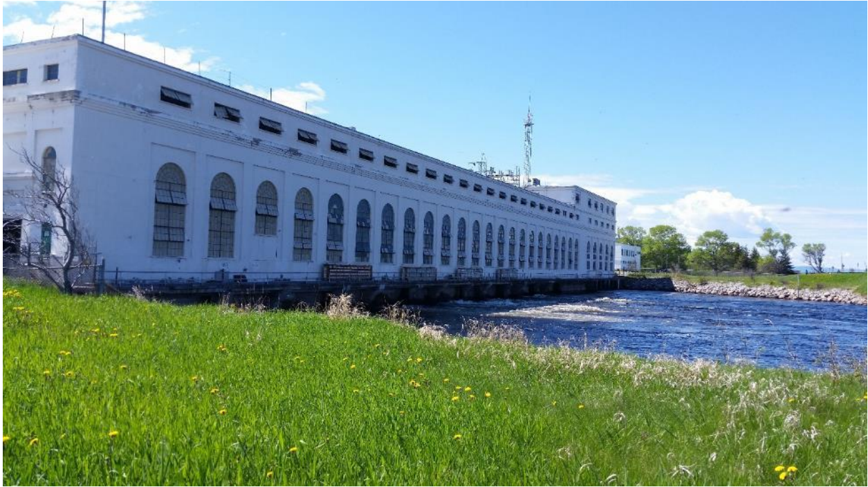
The Powerhouse (hydroelectric plant) in Deer Lake, June 2016
